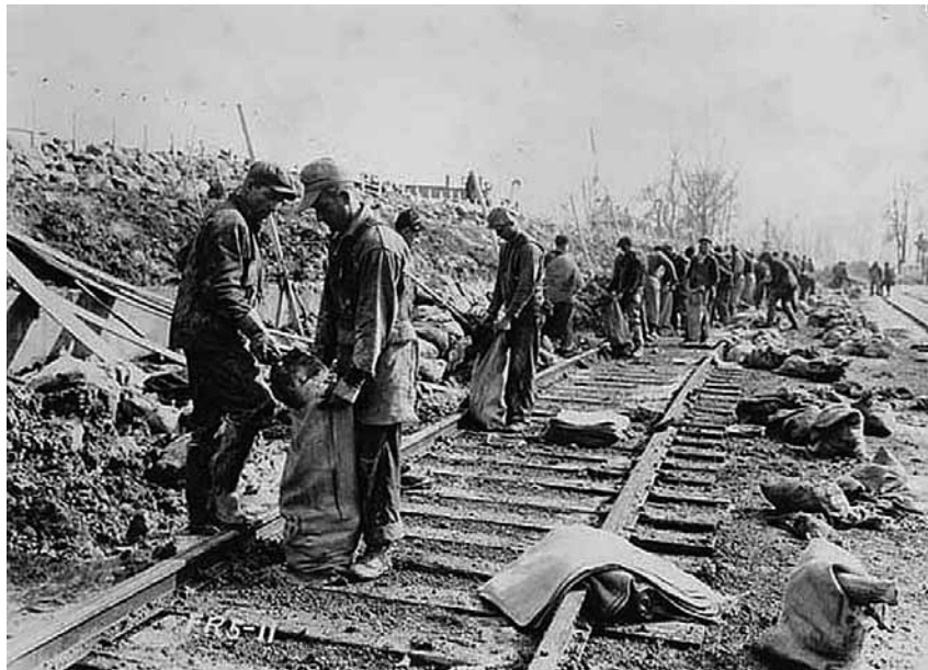
In Cairo, Corps men filled sandbags for flood control. Photo courtesy of the Abraham Lincoln Presidential Library and Museum.
